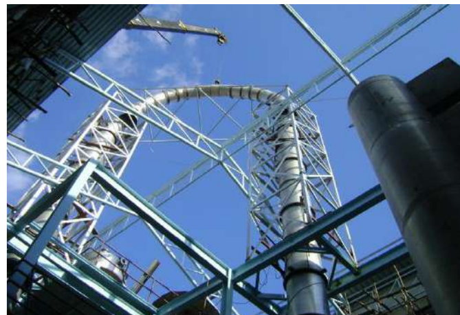
Cyclone construction for use in flour transportation systems
