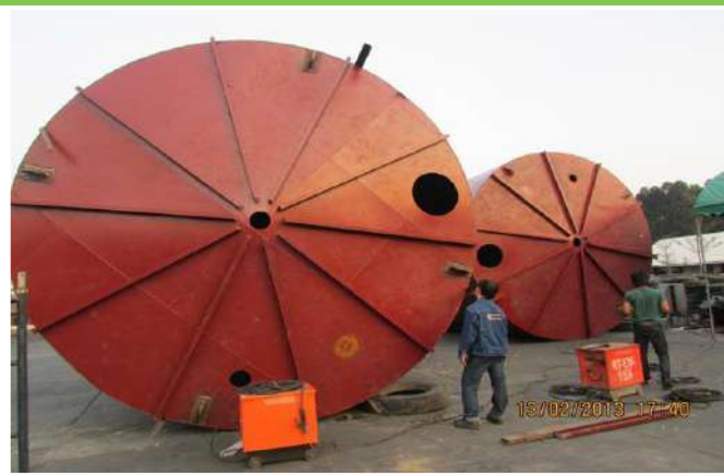
Construction of 120 cubic meters of carbon powder storage silo
