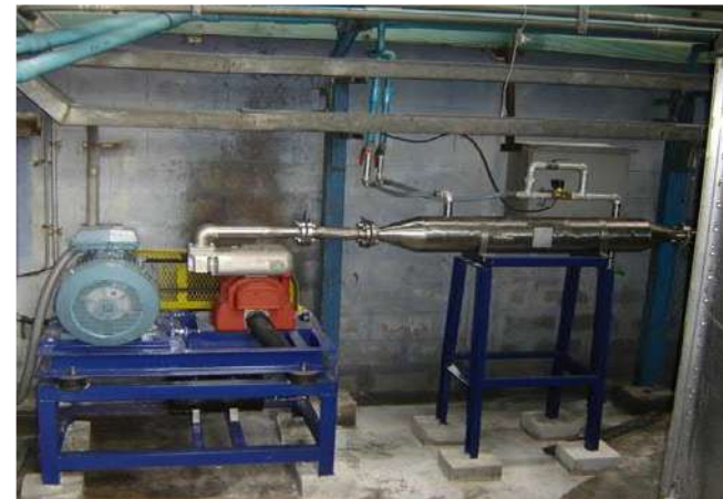
Plastic pellet transportation system from sea bulk cars up to Silo
