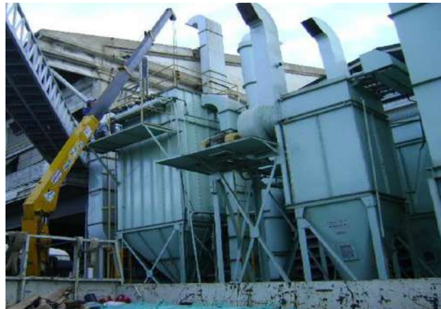
Piping system, absorbing carbon powder
