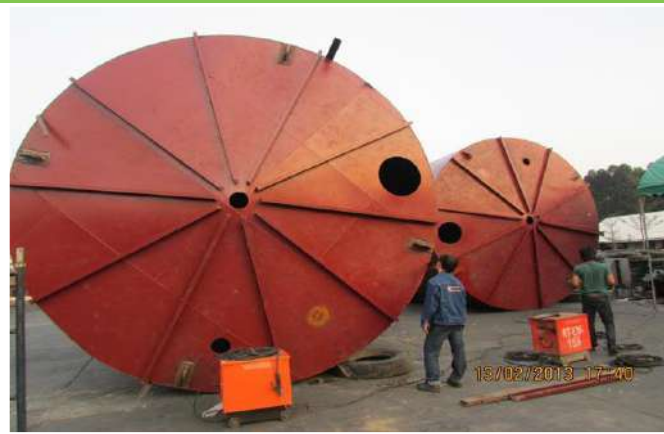
Construction of 120 cubic meters of carbon powder storage silo
