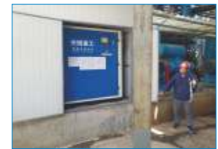
A Thermal Power Plant in Gaomi
