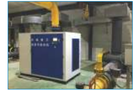
A Sewage Treatment Plant in Chongqing
