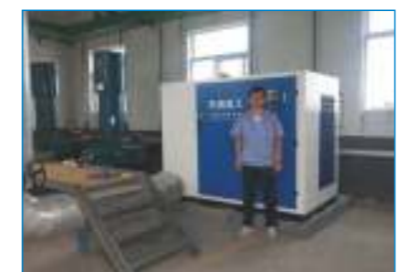
A Sewage Treatment Plant in Shouguang
